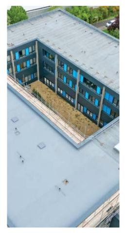
Image above courtesy of Rooftek Advance Ltd, Reading: Single ply membrane roof refurbishment at Broadwater Apartments, Worthing.
